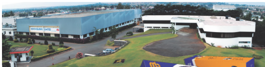
Menon Bearings plant at Kolhapur,
