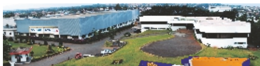
Menon Bearings plant at Kolhapur,
