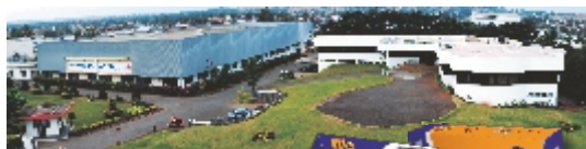
Menon Bearings plant at Kolhapur,
